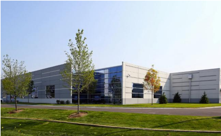
Curtain wall and pre-cast concrete panels façade Building CH2, Elk Grove, IL
