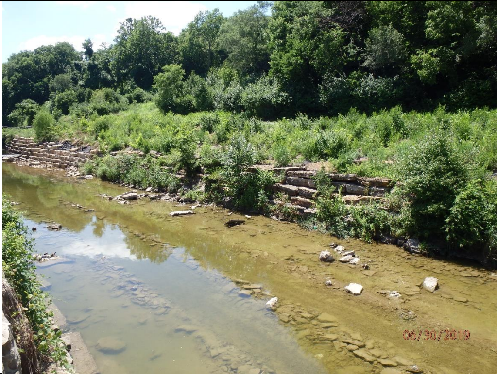
I – REPAIR WALL - $110,000
