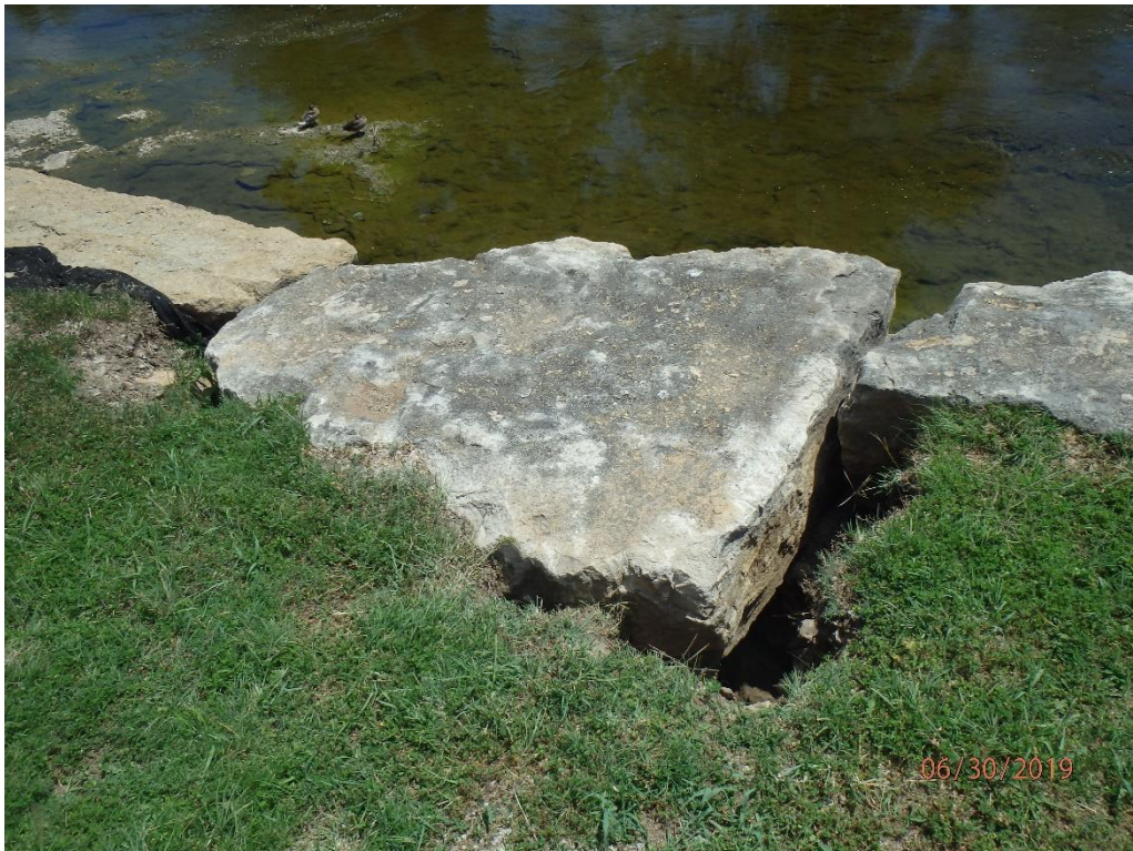
A – HOLE REPAIR - $500
