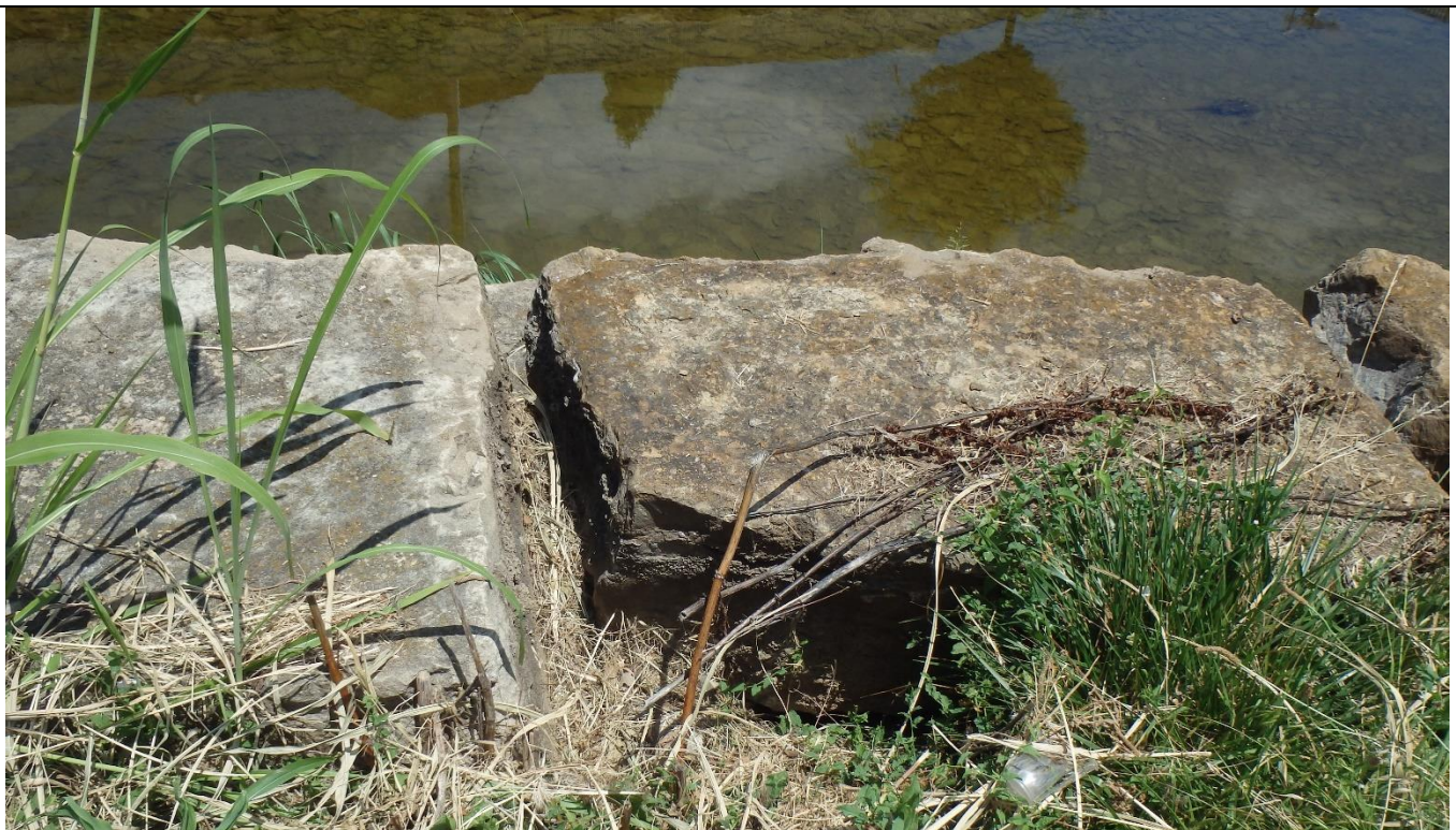
H – HOLE REPAIRS - $1,500
